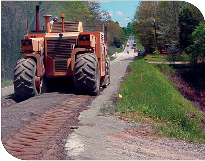
Recycling old asphalt pavement using FDR.
