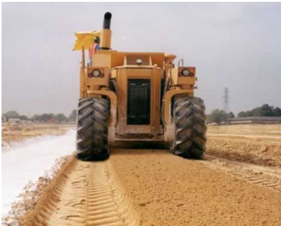
Figure 14: Rotary mixer used for initial mixing
